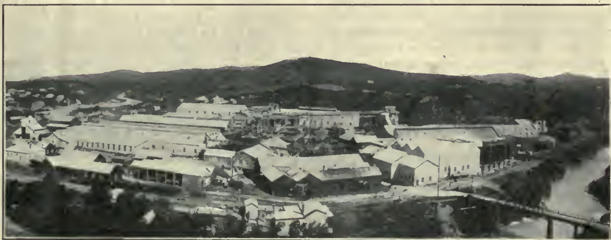
Waihi company's 200-stamp mill, sand, slime, and concentrate treatment plants at Waikino, 6 miles from the mine. Power used is water, steam, gas, and electric. Transmission lines from the hydro-electric plant cross the hills at the right. The highest peak showing is Mt. Te Aroha, 3120 ft. Ohinemuri river in the foreground. This is used for water power and as a 'sludge-channel' for residue from all mills in the Waihi-Waitekauri-Karan-Gahake districts.
